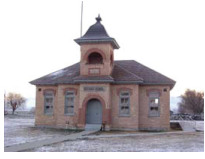
Fairfield School House, 1898
