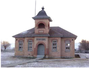
Fairfield School House, 1898
